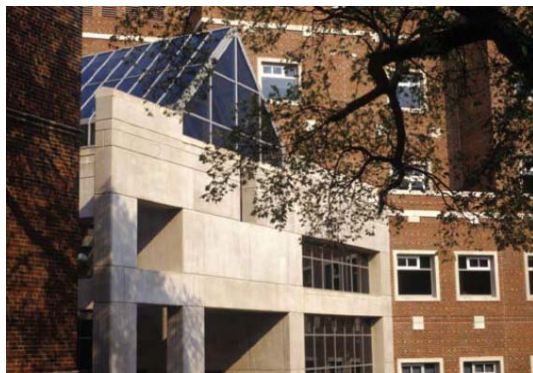
The Science and Engineering Research Facility (SERF)
